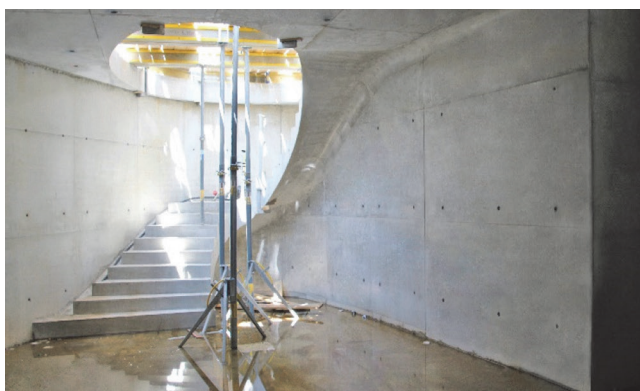
Figure 6. Appearance of the staircase after removing the 3D printed formwork [31]
